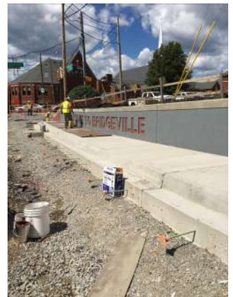
Widening of Chartiers Street, new Welcome Wall
