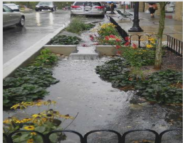
Example of stormwater control measures in State College, PA
