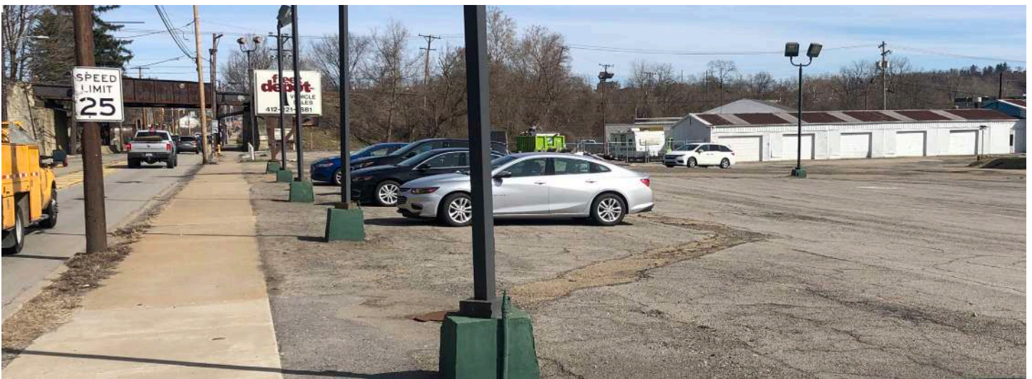
Existing conditions along northern end of Washington Avenue, Photo Courtesy of Mackin
