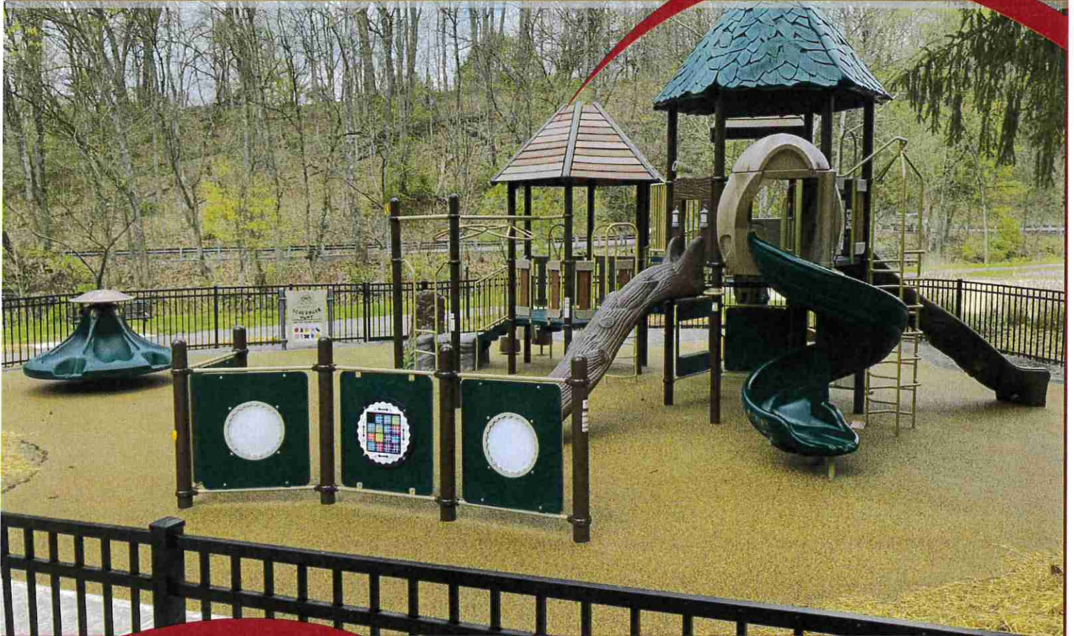
McLaughlin Run Park—New Playground, Construction Completed
