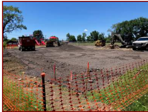
Project Construction Photo — July 9, 2024
