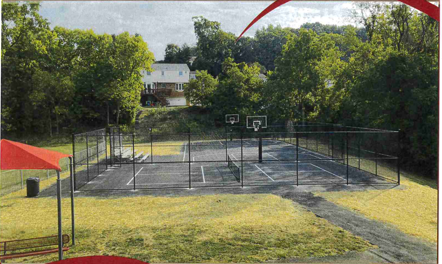
Cook School Park Basketball and Pickleball Court Renovations Completed
