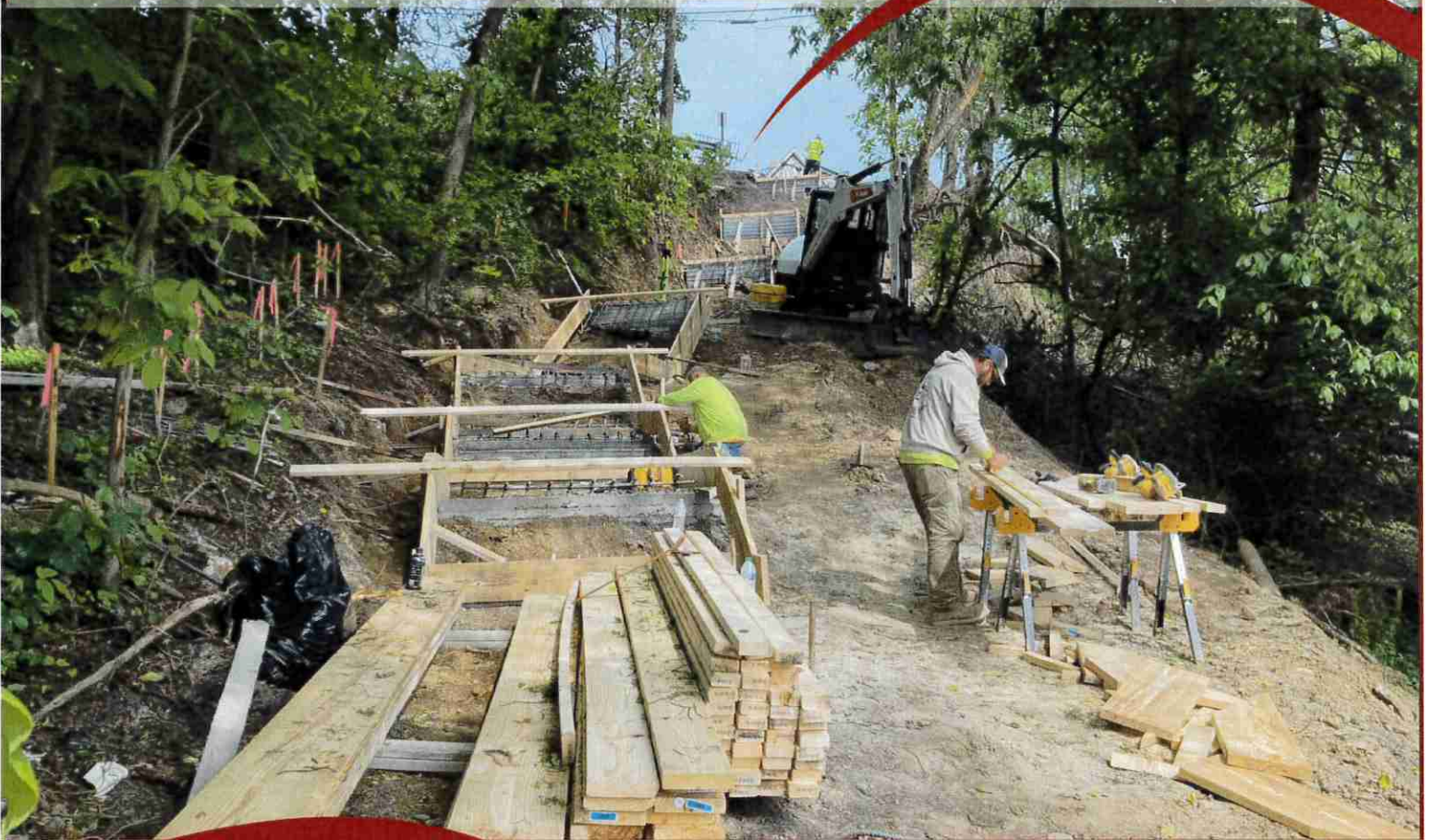
Gregg Ave. Steps Construction Project—Progress Photo, May 2025
