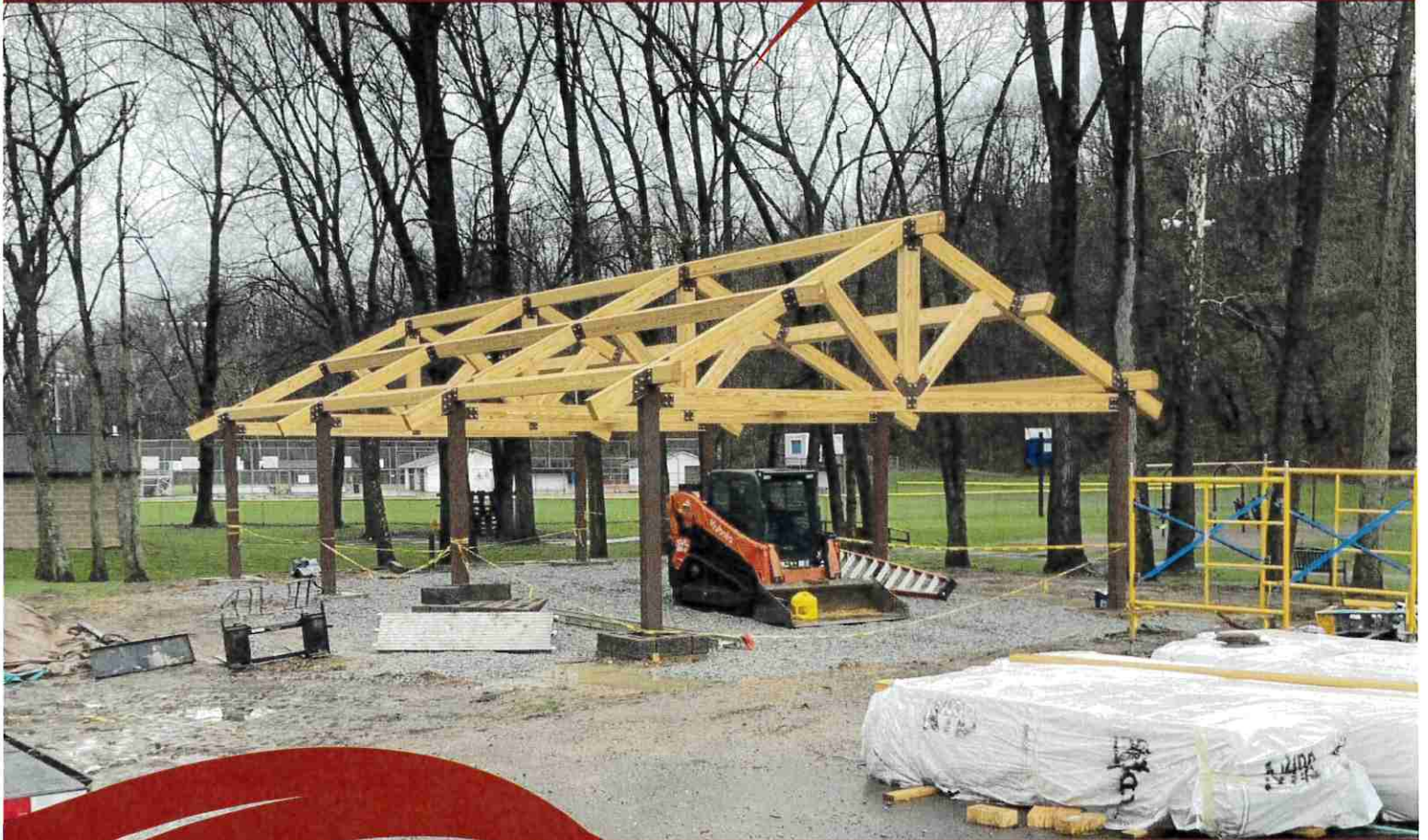
New Chartiers Park Shelter No. 1 Under Construction
